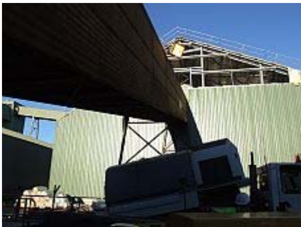
Figure 1.8 Exterior view of conveyor 21
