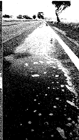
Bruce Rock to Shackleton Road “Upgrades” have subsided and are quickly deteriorating.
