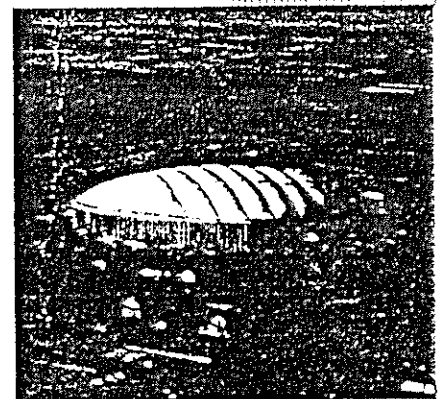
The economy of air-supported structures is demonstrated by the UNI-Dome covered sports stadium. Total cost: $7 million.
