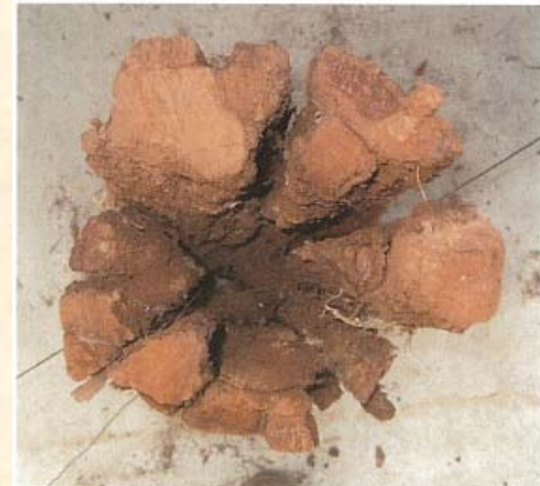
Picture 6. Pole PID# 338952 showing extensive decay and sectionalisation
